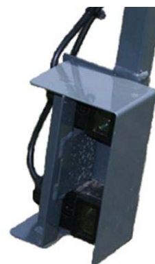
Photo Light Sensor -Typical View
