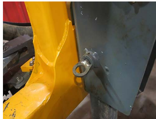
Lock Pin Removed -Typical View
