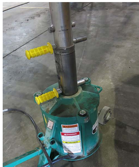
Lock Pin Installation -Typical View
