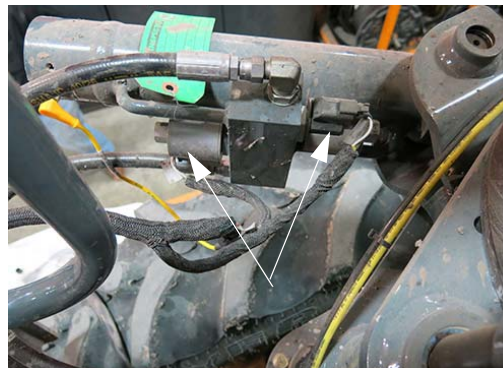
Lock Valves -Typical View
