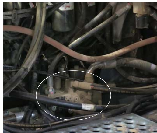
Hydraulic Valve Block (Located near the rear right-hand service platform - open hood to access) -Typical View
