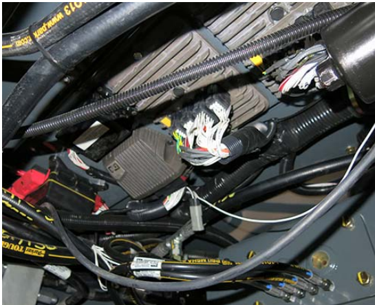
Circuit Breakers/Fuses (Exterior) (Located beneath cab - remove panel to access) -Typical View
