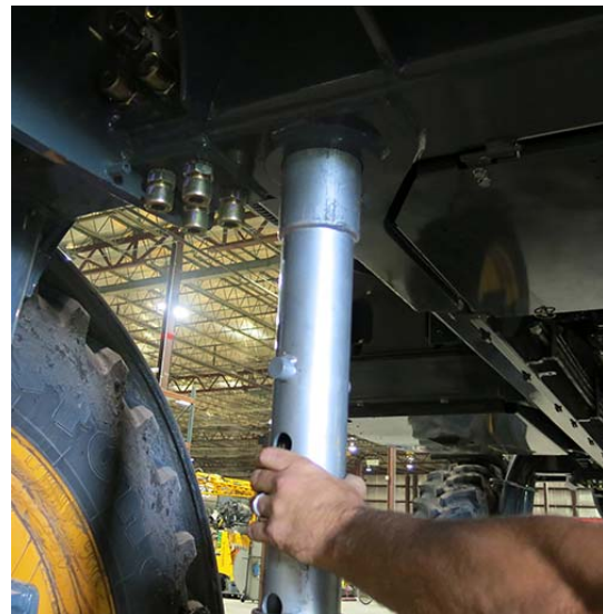
Insert Jack into Lifting Point Containment Ring -Typical View
