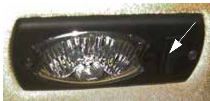
Interior Work Light Switch -Typical View
