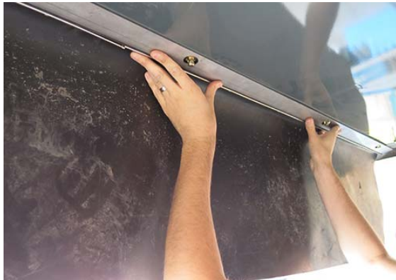
Brush Curtain Installation -Typical View
