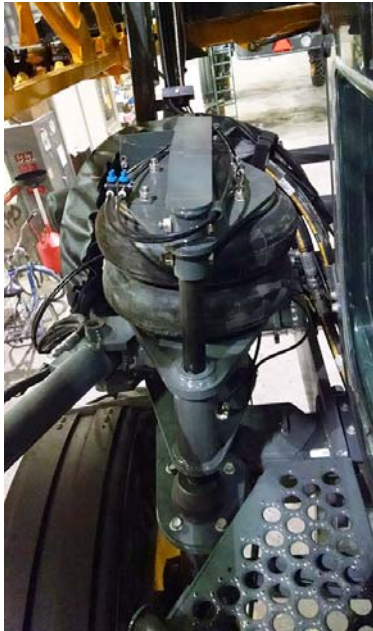
Air Bag (Located on each leg) -Typical View * Front Air Bag Shown
