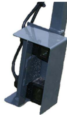
Photo Light Sensor -Typical View
