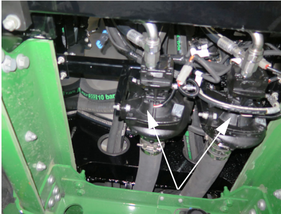
A - Solution Pumps
