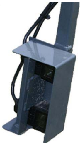
LS Photo Light Sensor Assembly -Typical View
