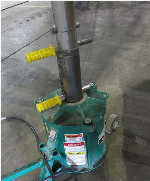
Lock Pin Installation -Typical View
