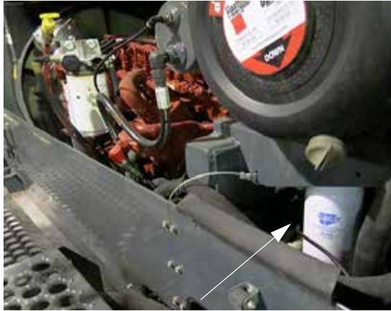
Hydrostatic Charge Pressure Filter (Located behind left-hand engine compartment) -Typical View
