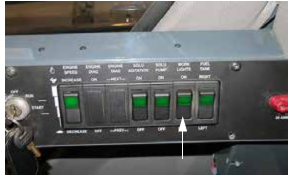
Work Lights Switch (Located on side console) -Typical View
