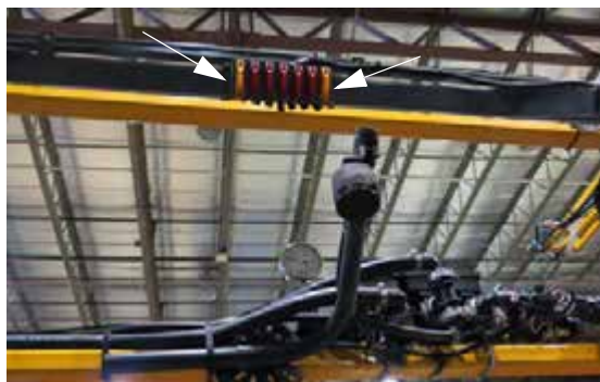
Fence Row Indicators (Located on transom) -Typical View
