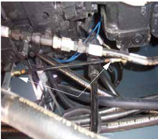
Hydrostatic Pump Controller -Typical View
