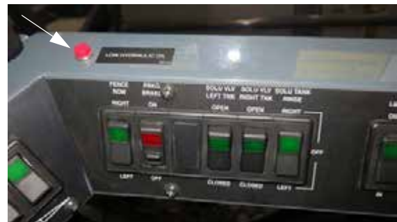
Low Hydraulic Oil Indicator (Located on the side console) -Typical View
