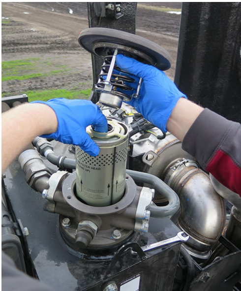
Return Filter 1 (Located inside filter housing) -Typical View
