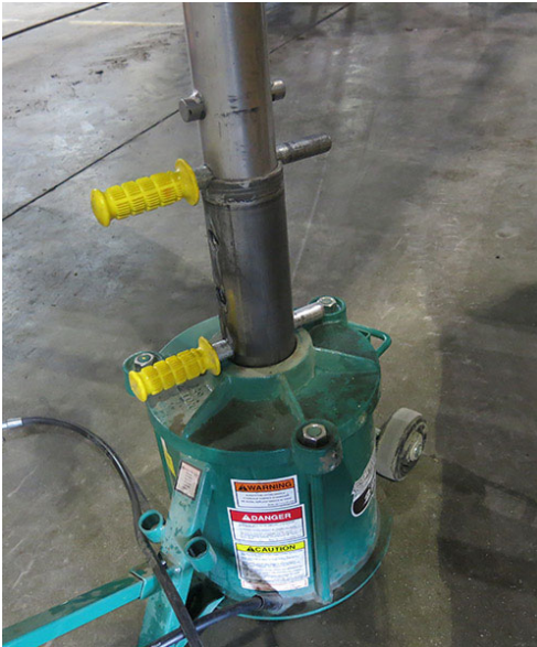
Lock Pin Installation -Typical View
