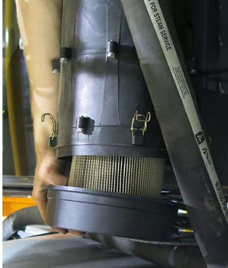
Filter Removal -Typical View
