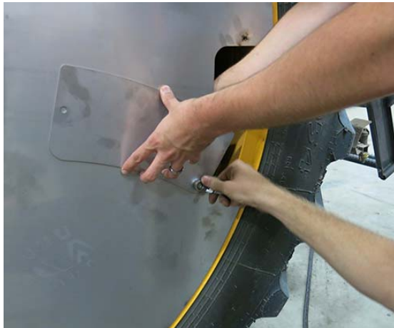
Valve Stem Access Panel -Typical View
