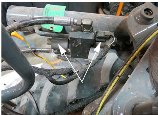
Lock Valves -Typical View
