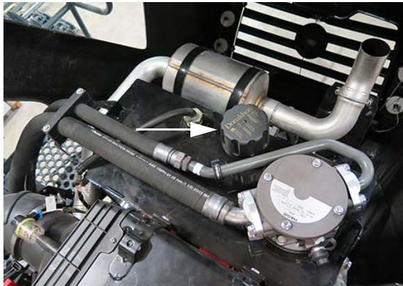
Tank Breather Cap (Located on top of hydraulic oil reservoir - open hood to access) -Typical View
